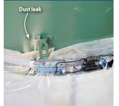
Band clamps don't always form a tight seal when securing a bag, which is usually oversize, to the machine's rim, creating a dust leak under pressure.
