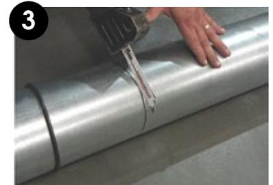
3 Use O-ring (comes with nipple) to mark cut line. Cut.
