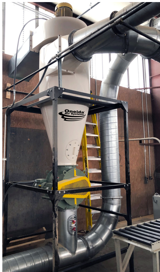
Oneida Air Systems' 20HP Direct Drive Dust Collector installed at Trimjoist's facility.
