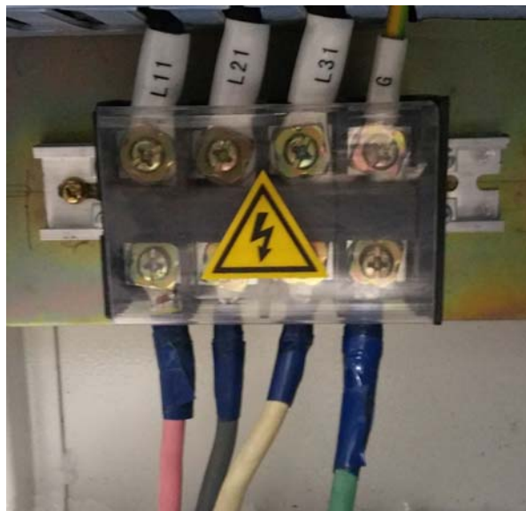
Fig. 1.6 Main power connection.
